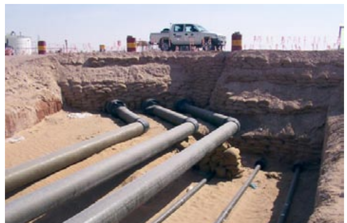
Fig. 6.5. Main assembly inside the trench
