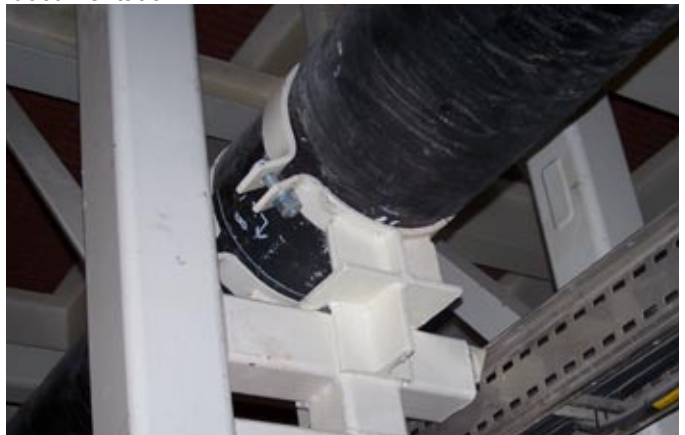
Fig. 7.4. Support with fixed point
