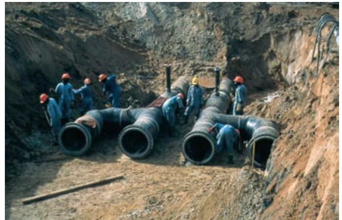
Fig. 6.8. Pipe assembly in process in prepared trench
