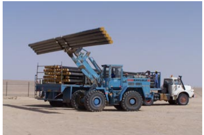
Fig. 3.3. Pipe handling (unloading)
