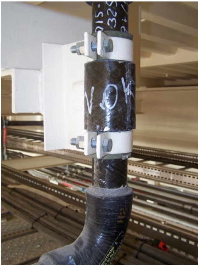
Fig. 7.5. Fixed point with bonded saddles
