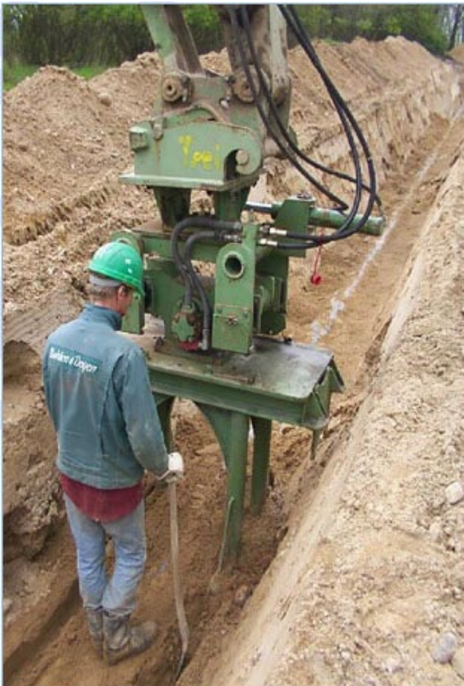
Fig. 6.9. Compaction of backfill material
