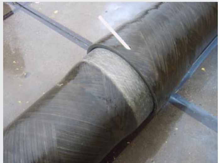
Fig. 4.8. Mechanical O-Ring joint (1-key)
