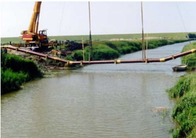
Fig. 6.12. Lowering underwater main
