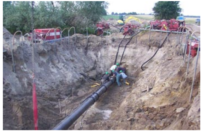
Fig. 6.4. Assembly in process
