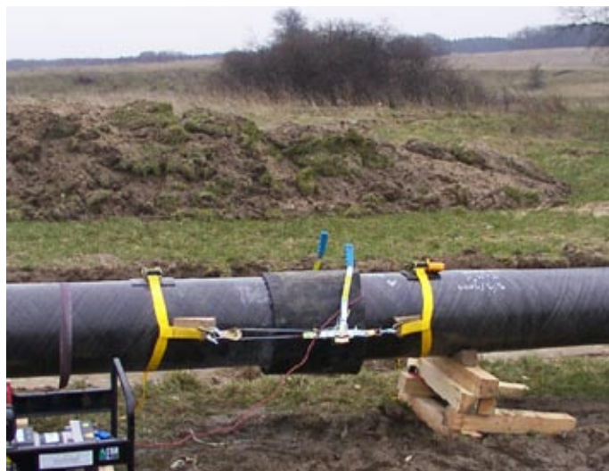
Fig. 5.5. Pulled adhesive joint
