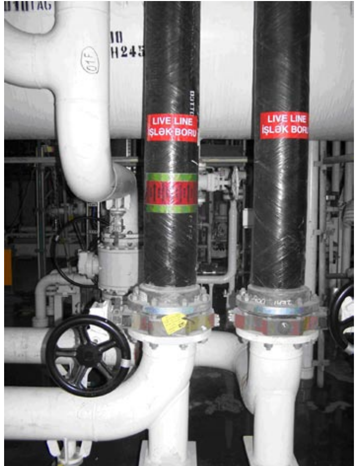
Fig. 7.16. Joining to other materials
