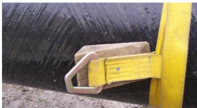
Fig. 5.7. Wedge between pipe and pulling lug
