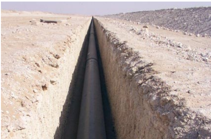
Fig. 6.2. Trench in stable soil
