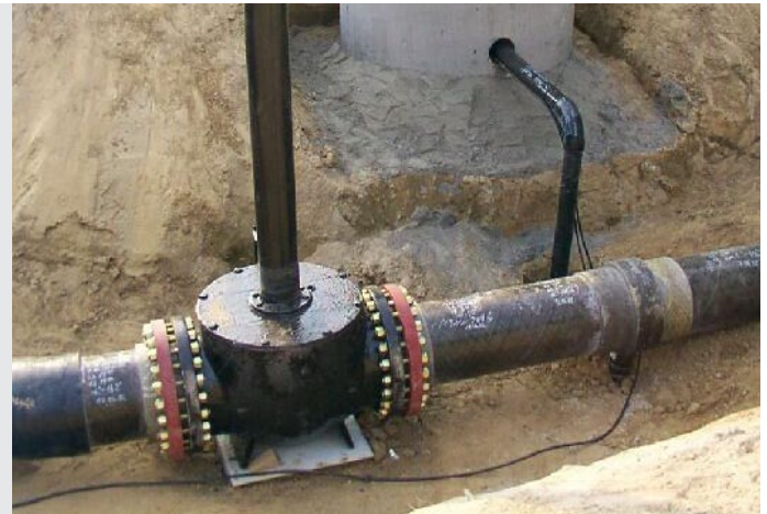
Fig. 4.5. Flanged joint
