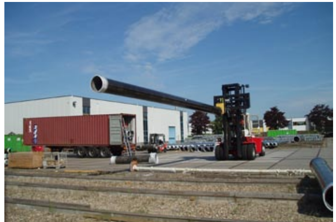
Fig. 3.4. Pipe handling (loading)
