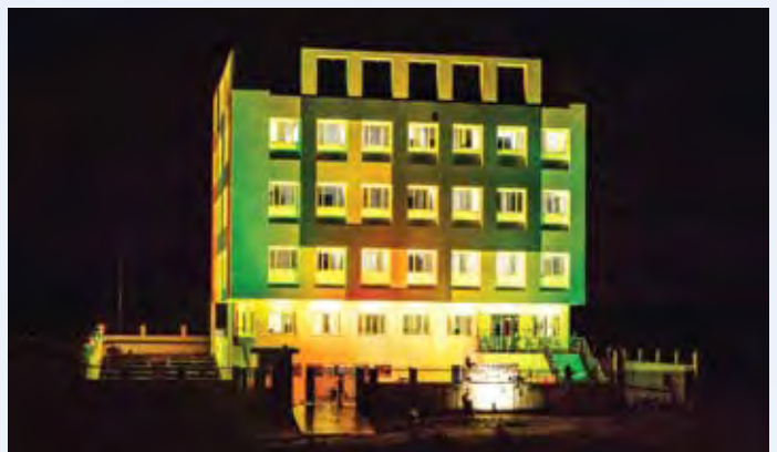
Vocational cum skill development centre at Udaipur
