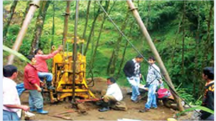
Exploratory drilling for Geotechnical investigations for Bhanupali-Bilaspur-Beri New BG Rail Link
