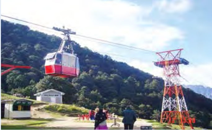
Revamping of Ropeway at Joshimath-Auli
