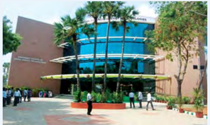
Green Building of Madanjeet school of Green Energy Technologies (MSGET) for Pondicherry University at Pondicherry
