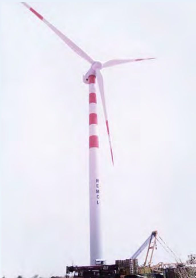
Wind Mill project of Railway Energy Management Company Ltd (REMCL)-under installation
