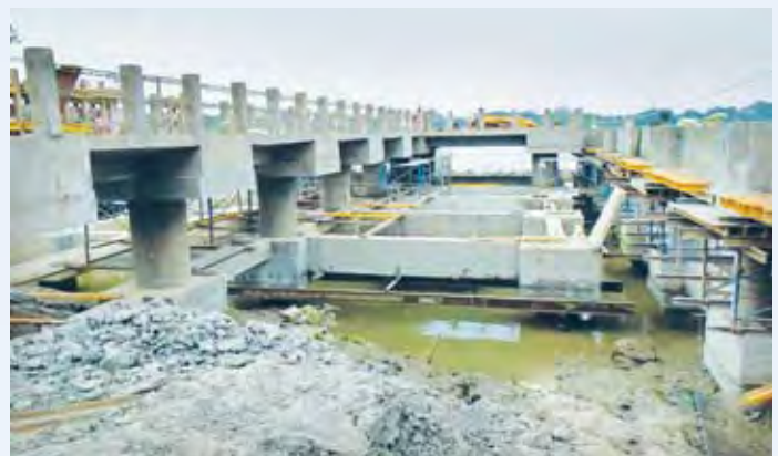
Raw water intake Jetty construction, Ma-er-Ghat, Baghbazar, Kolkata
