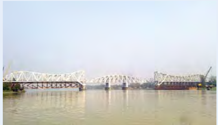
Three Span Continuous(132.65m+150m+132.65m) Railway Bridge Across River Hooghly on Naihati – Bandel section of eastern Railway, near Kolkata (West Bengal) in Replacement of existing Jubilee Bridge
