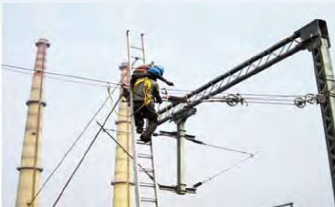
Railway Electrification work at Rourkela Steel Plant Railway Siding
