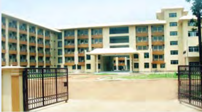
Construction of 2000 Bedded Hostel for Boys at IIT Kharagpur, West Bengal.
