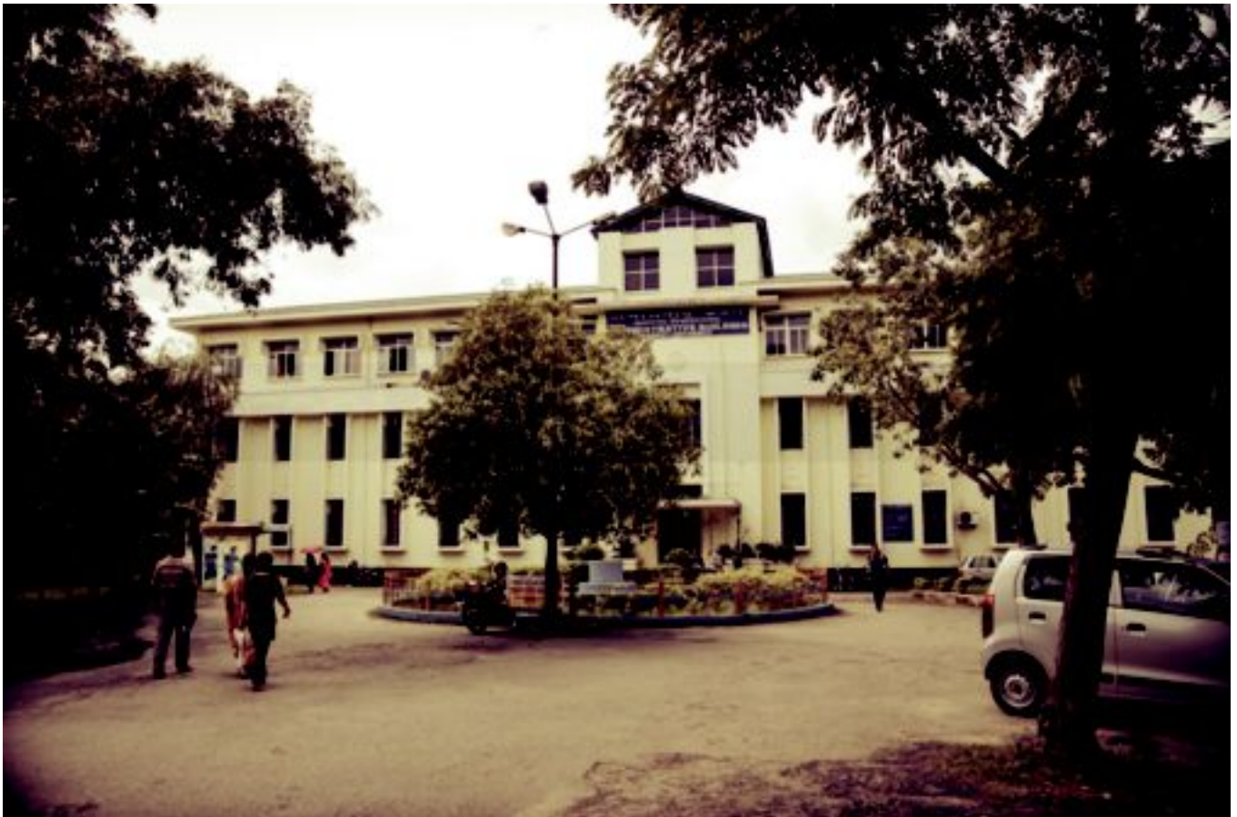
A view of the Administrative Building, G.U.
