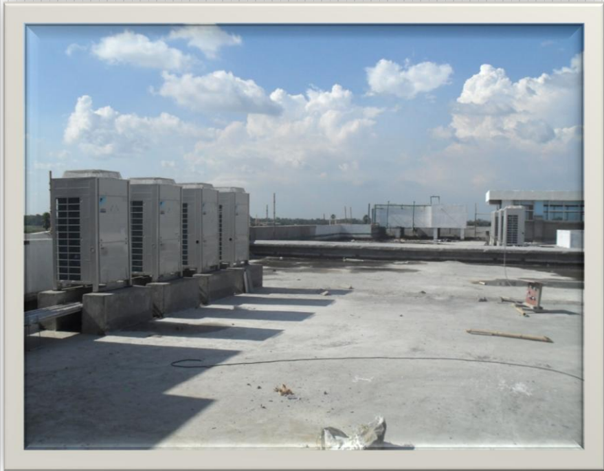
HVAC OUT DOOR UNIT AT ROOF
