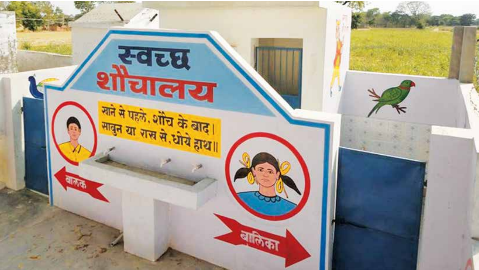
A beautifully designed toilet infrastructure built by Panchayats in Mirzapur district, Uttar Pradesh
